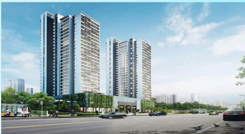
KHU CĂN HỘ PARK VIEW RESIDENCE P. THANH MỸ TÂY - TP. HCM
